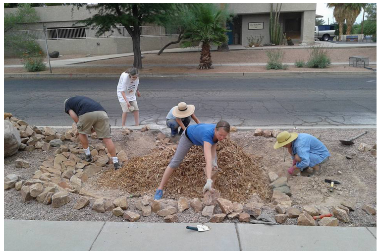
A level tree terrace is being created on the right side of this basin. Rock is used to stabilize the lower and upper edges of the terrace.
