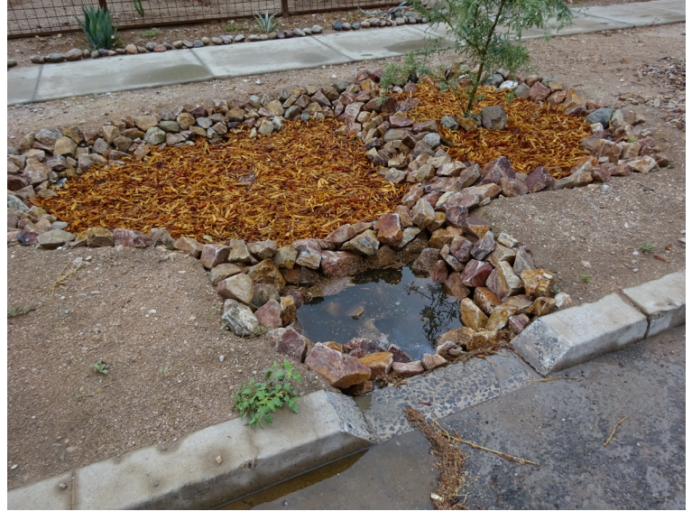
The sediment trap collects debris while still allowing water to flow into the rest of the basin.
