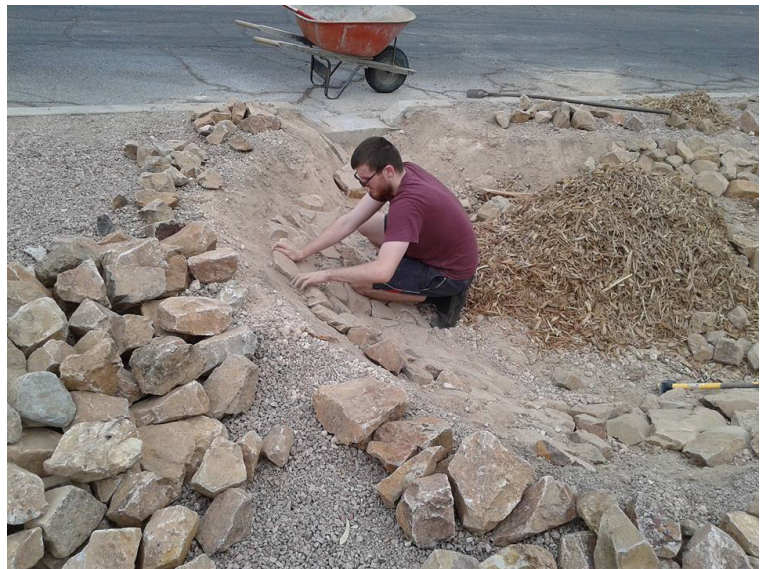
Fit rocks together like a jigsaw puzzle, using the lower course of rocks to serve as an anchor for the next row.
