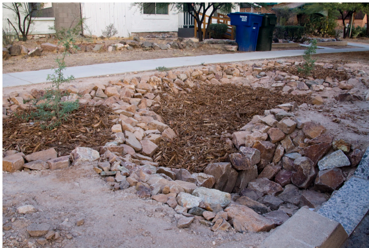
Trees are planted on terraces slightly higher than the bottom of the basin to prevent their trunks from being submerged in water.
