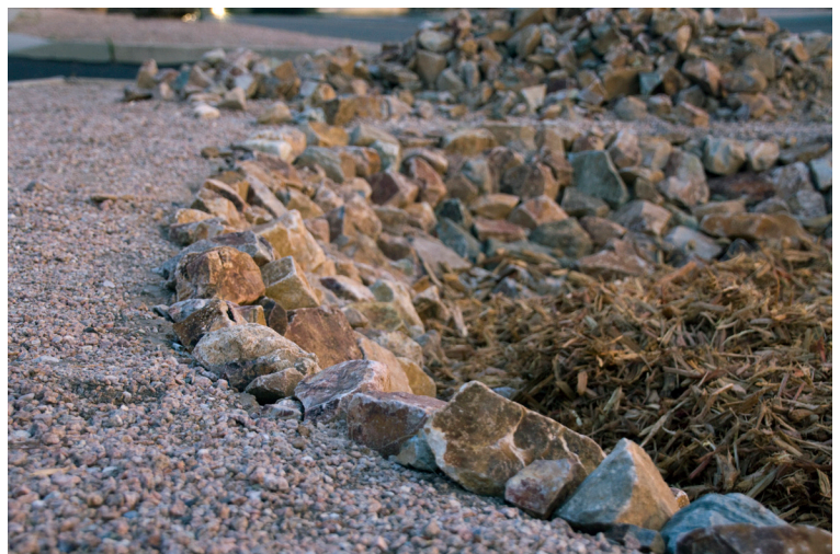
The top row of rocks is above the level of ground surrounding the basin. Water will still make its way into the basin, but this prevents erosion of soil and gravel into the basin.
