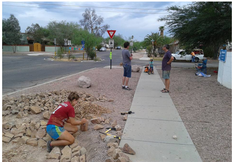
Start by placing large anchor rocks in a shallow trench along the base of your basin slopes.
